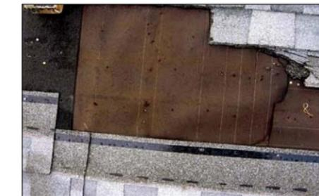
Blown-off shingles may expose your home to structural damage, mold, and mildew.
